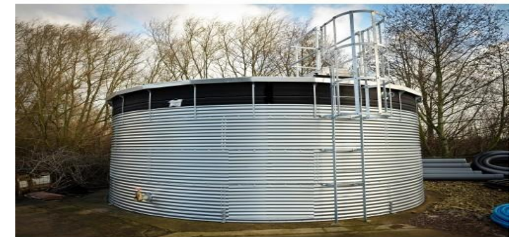
G.I Pre-fabricated Water Tank with PE Lining
